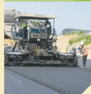
| Placement and Compaction |
