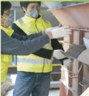
| LEADCAP Additive Added into Plant Mixer or Asphalt Tank |
